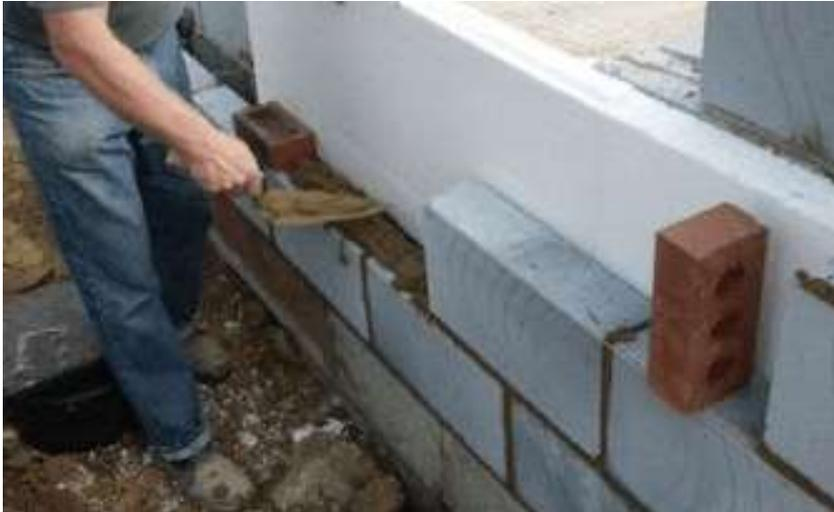
Two leaves should be constructed simultaneously. Spacing should be uniform and it is attained by predetermining the location of wall ties. Damp proof course is provided for two leaves separately. In case of doors and windows, weep holes are provided above the damp proof course.
