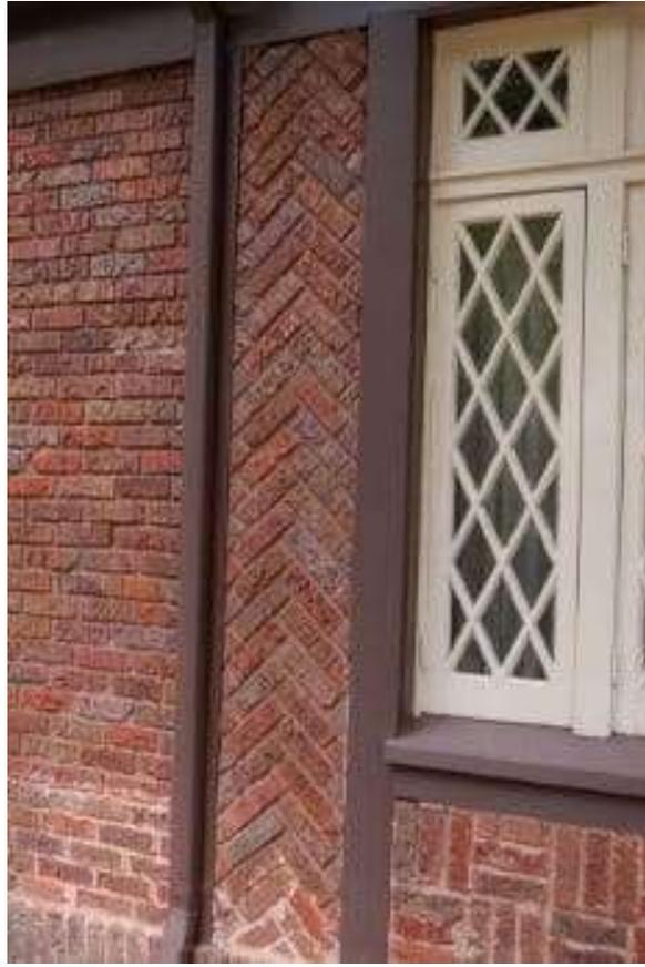
Fig. 5: Brick nogging partition wall; bricks are laid on edge
