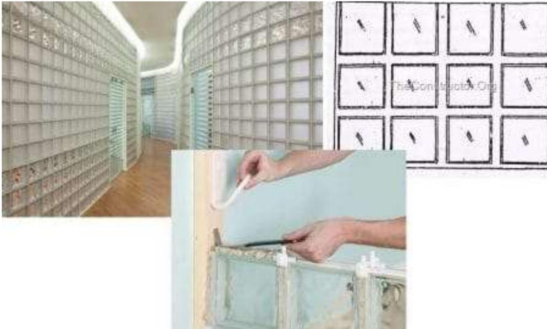
Fig.9: Glass block partition wall
